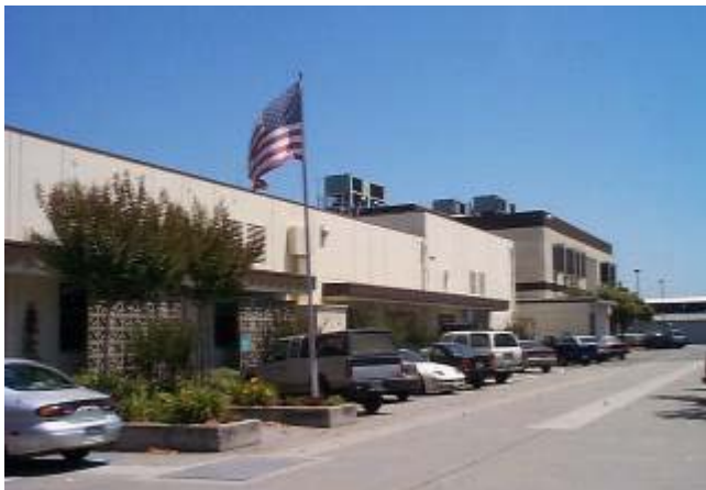
Existing Laboratory Remodel
