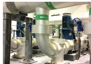
Dubai South District Cooling, Dubai,
