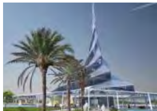
Solar Innovation Center, Dubai
