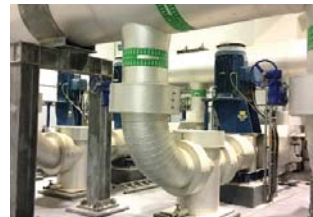
Dubai South District Cooling, Dubai,
