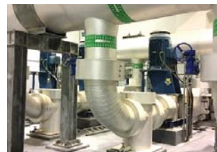
Dubai South District Cooling, Dubai,
